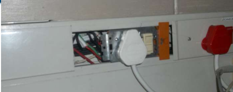
No covers for the socket outlets on power skirting.
