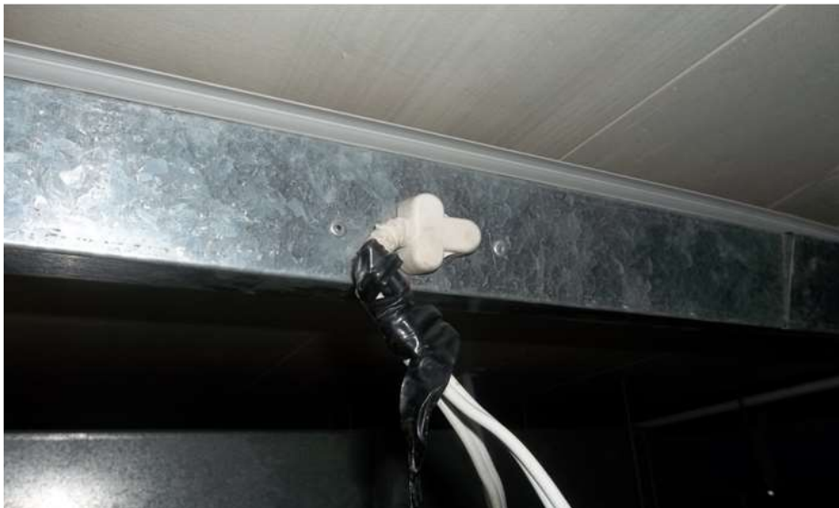
Multiple lights sharing a 5A plug. Improper joints were done.
