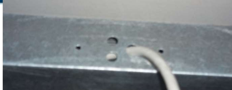
Cable connected directly into the P8000 wire way instead of through a socket outlet.
