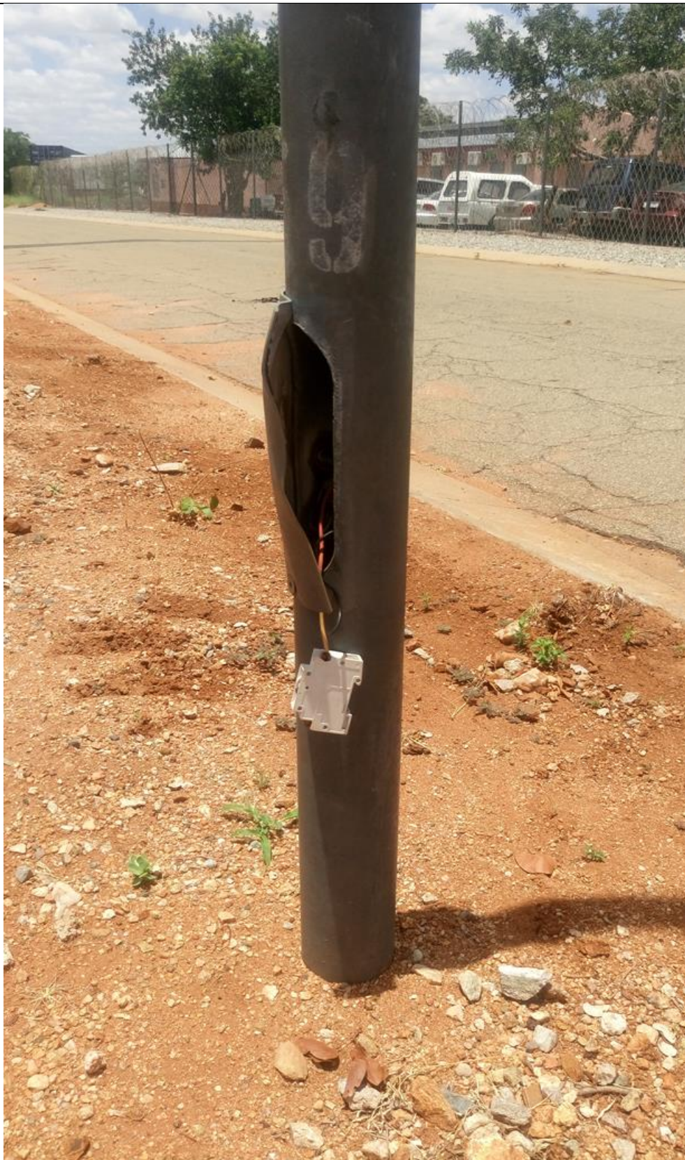
Figure 03 Vandalised Control Circuit of Streetlight
