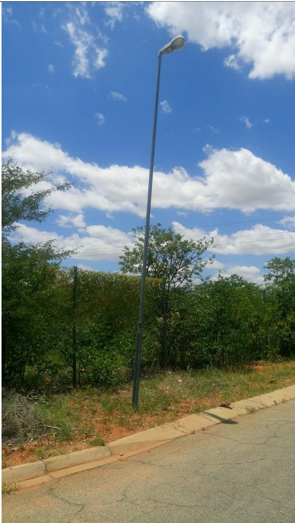
Figure 05 Skew Existing Streetlight Pole
