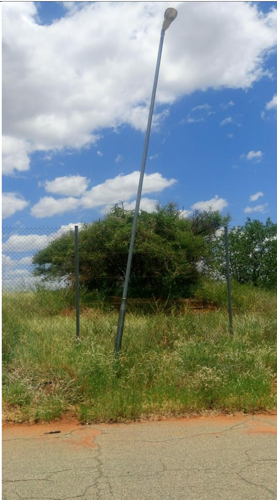
Figure 02 Existing Vandalised Streetlight Pole
